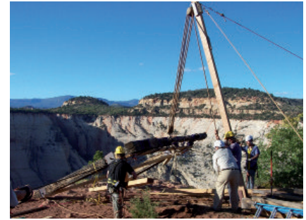
Figure 10: Workers use a traditional gin pole with a block-and-tackle to lower the front bent of the Draw Works. Workers, when in proximity to the cliff edge, wore harnesses and were securely belayed. Photo Credit: University of Vermont
