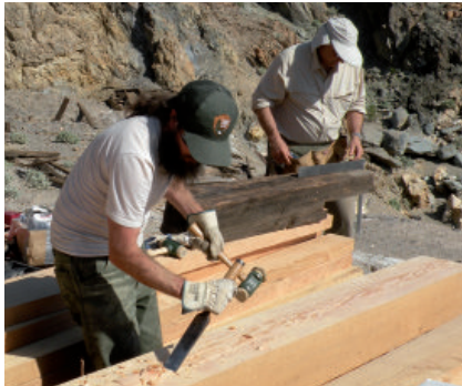
Figure 5: Death Valley National Park employee Jeremy Stoltzfus uses mallet and chisel to properly size a replacement timber. Timber framer Mike Controneo works on a scarf joint in the background.
