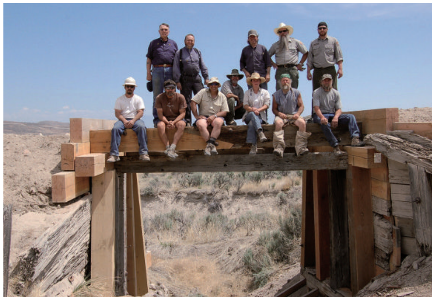
Figure 16: Crew members, including students, park staff, and timber framers, pose with principal investigator Doug Porter (third from right, back row) on the rehabilitated trestle. Note the scarf joint joining new and historic material on the front stringer. Photo Credit: Holly Strachan
