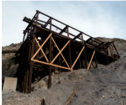
Figure 6: New diagonal bracing, with repairs to posts, ensures that the lower terminal will remain standing.
