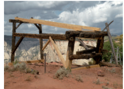
Figure 12: The rehabilitated Draw Works. Only members deteriorated beyond repair were replaced. Where possible, splices joined sound historic material to new replacement wood to retain as much original material as possible. Photo Credit: Randall Skeirik
