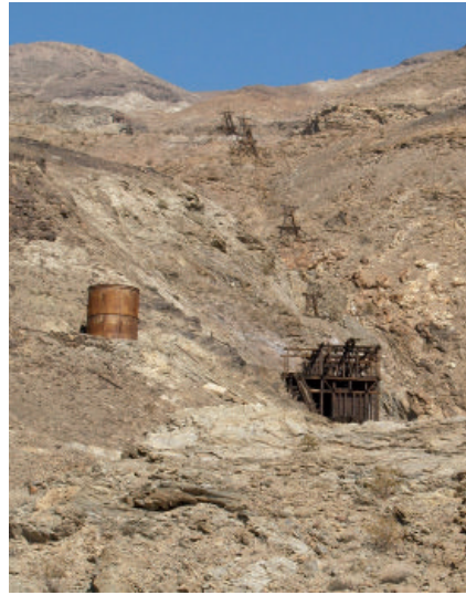
Figure 3: The Keane Wonder Mine tramway, with lower terminal and the first six of its 11 remaining towers. Photo Credit: Randall Skeirik
