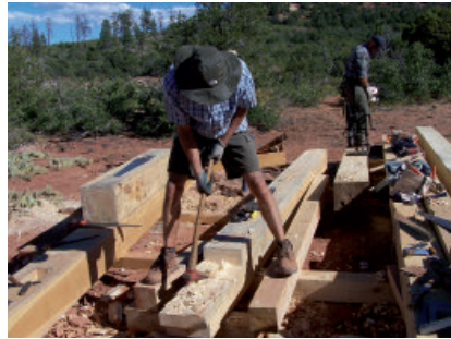
Figure 11: A volunteer learns how to use an adz to shape a timber. Photo Credit: University of Vermont
