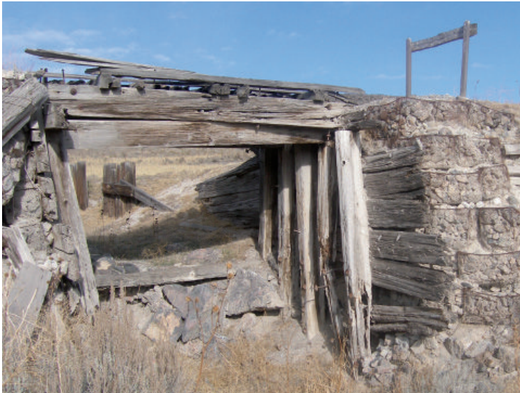
Figure 13: Trestle One, with severely deteriorated east-bent posts, failing head wall and stringers. The stone gabion baskets were installed by the National Park Service in an earlier stabilization effort. Photo Credit: Randall Skeirik
