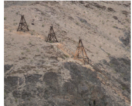
Figure 7: Tower 7 (at right), on the edge of the canyon, was about to collapse. Assessment of each member led to replacement of only those members or portions of members too deteriorated to be repaired. One of the last remaining ore buckets hangs between Towers 8 and 9. Photo Credit: Randall Skeirik
