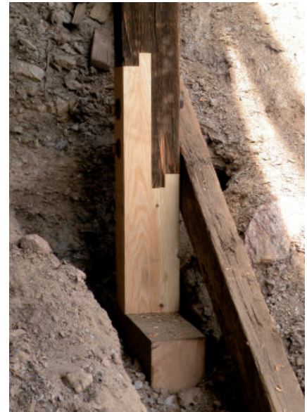
Figure 4: In keeping with preservation philosophy, only the deteriorated portions of framing members were removed. The bottom end of this post has been replaced with new, matching material. This splice joint was laid out and cut by the VT historical architect under the supervision of a timber framing expert. Photo Credit: Randall Skeirik
