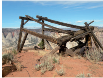
Figure 9: Upper terminal of the Cable Mountain Draw Works prior to preservation. Note the deteriorated corner post, which causes the structure's forward lean, and cable looped around the structure to prevent it from tumbling over the cliff should it collapse. Photo Credit: Randall Skeirik
