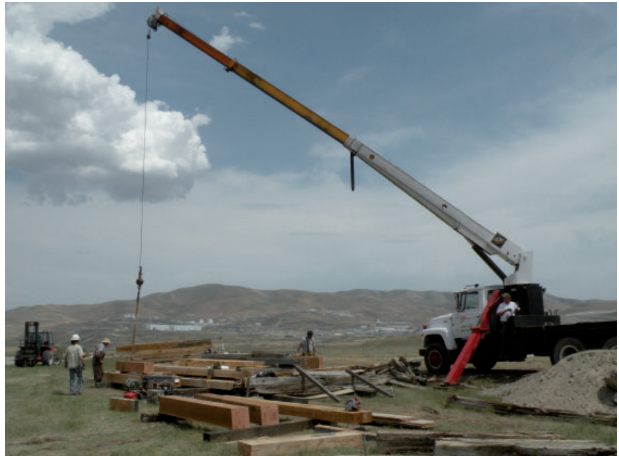
Figure 15: Stockpiled timbers at the site of Trestle One. The crane is about to lift a replacement post into place. Photo Credit: Randall Skeirik
