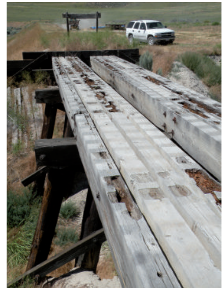
Figure 14: Trestle Two, showing creosote-treated posts and beams. The stringers that run the length of the trestle were not creosote treated and show significant deterioration that will require repair. Photo Credit: Randall Skeirik
