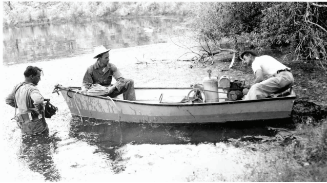
H.J. Charbonneau's dive. Note compressor and air reservoir in support boat. NPS photo by Park Custodian (Superintendent) Homer Hastings
