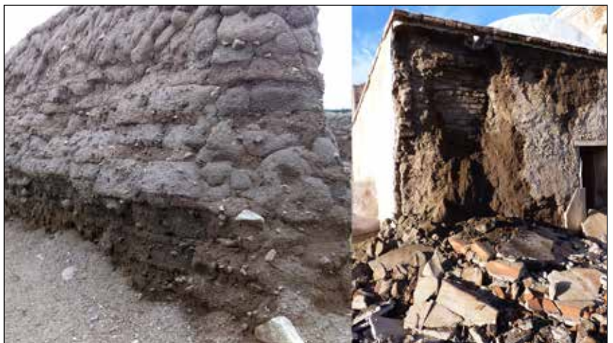
Figure 6. 6a (Left) Basal Erosion at Guevavi, Author, 2015; 6b (Right) Northeast sacristy wall collapse, Unknown, 2011, TUMA Archives.
