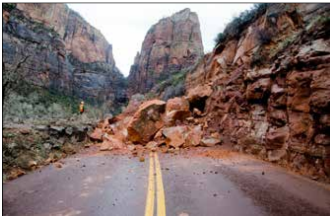
Figure 7. The rockfall that closed the Zion Canyon Road in January 2017, trapping 12 vehicles up-canyon. This rockfall—composed of large, sandstone blocks—occurred after a precipitation event due to undermining of the sandstone blocks, as identified in the initial USMP rating.
