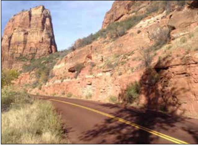
Figure 6. A photo of the slope that produced road-closing rockfall in January 2017. This photo, along with several others, was taken during USMP slope-rating activities and stored in the USMP database. The database identified this slope as unstable and prone to rockfall, with a potential failure mechanism of undermining as well as the presence of fractures to facilitate large-block release.
