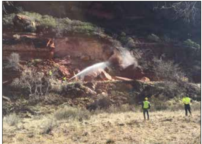
Figure 8. The successful use of a directed water jet to undermine two unstable sandstone blocks. The slope was permitted to dry for 24 hours afterward before crews could begin removing rock debris from the road below.
