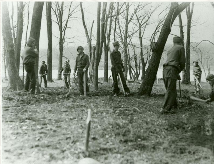
CCC workers clearing brush among trees at Theodore Roosevelt Island.
