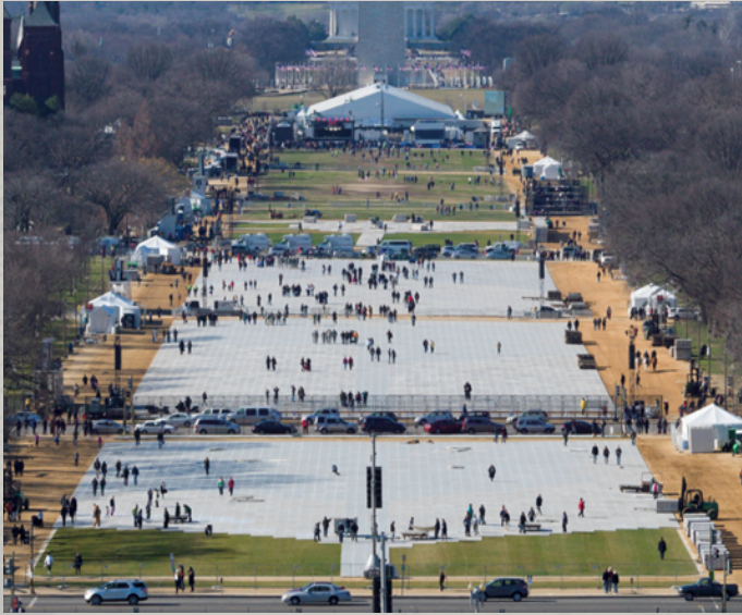
For the 2013 presidential inauguration at the National Mall park resource managers utilized polyethylene (HDPE) sheeting to protect the turf from extensive foot traffic (NPS).
