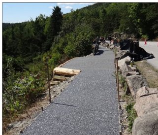
Filterpave on ACAD's Ocean Path.
