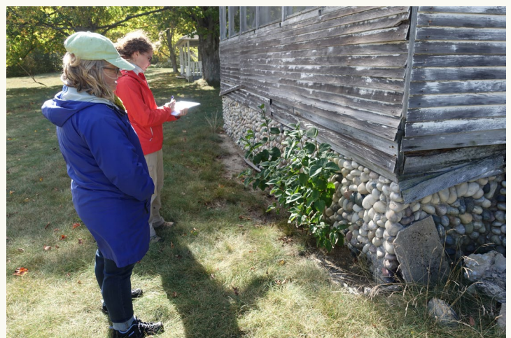
Volunteer lilac growing at the base of a stone foundation on North Manitou Island, SLBE.
