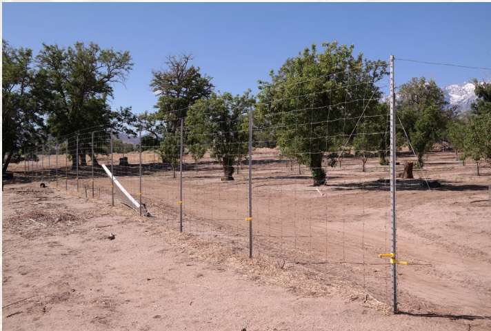
Deer resistant fencing with an electrified wire protects the historic Lydston orchard at Manzanar National Historic Site (NPS).
