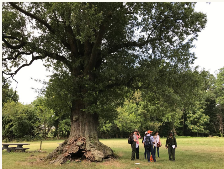
The 1812 Oak at Oxon Hill Farm at NACE has a deteriorating root ball and must be monitored for structural instability.
