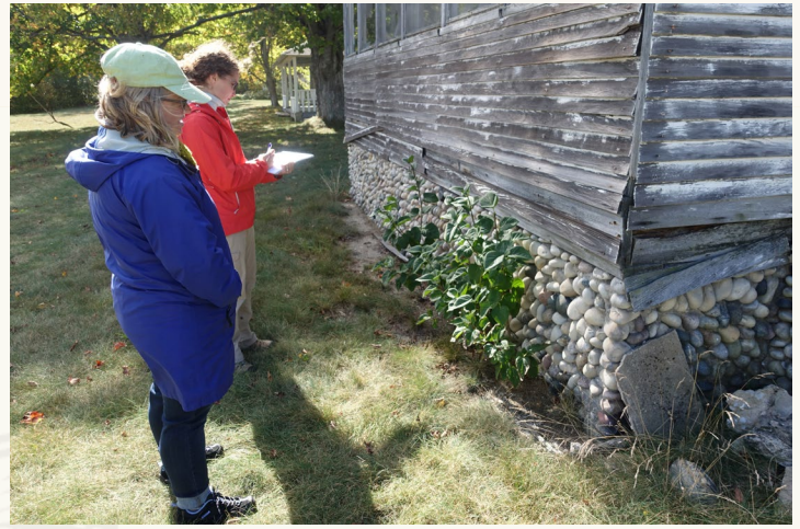
Staff evaluate a volunteer lilac too close to the foundation of a Cottage Row building on North Manitou Island at SLBE. A cutting can be taken and planted further out.
