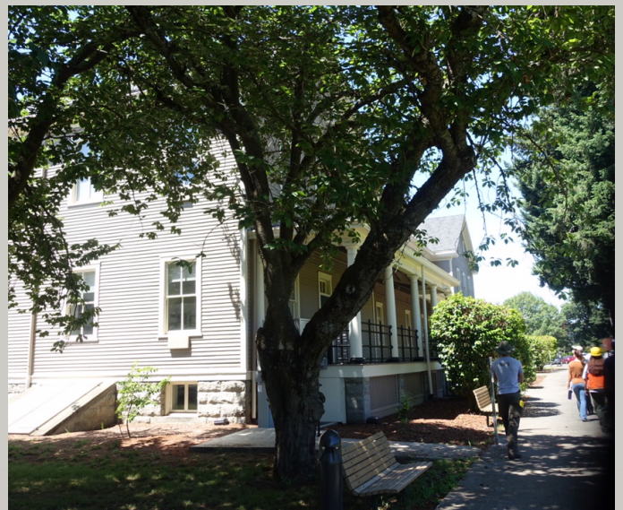
Formal military landscape at East Barracks. One of the areas that Brian helps to maintain (NPS).
