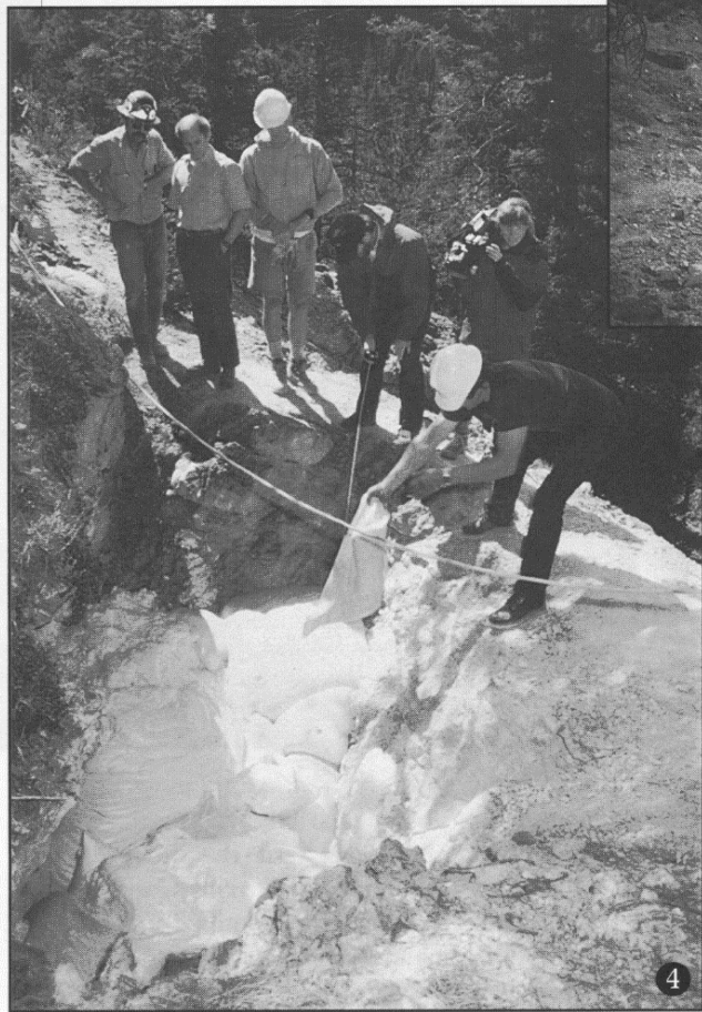
Figure 4. Installer directs expanding PUF foam into desired areas; Figure 5. The completed closure following earthen backfill.
