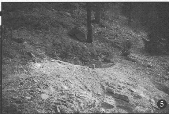
Figure 4. Installer directs expanding PUF foam into desired areas; Figure 5. The completed closure following earthen backfill.
