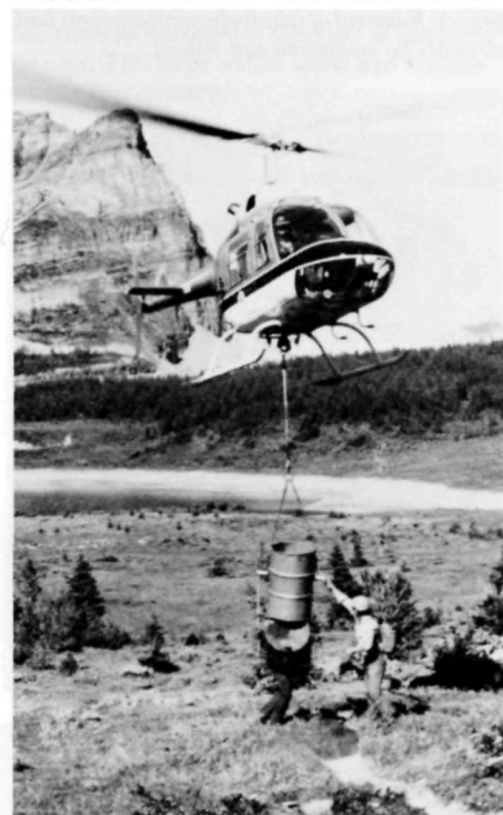
A specially modified common oil drum slung beneath the helicopter can carry 450 kg of fine gravel for maintenance and upgrading of trails.
