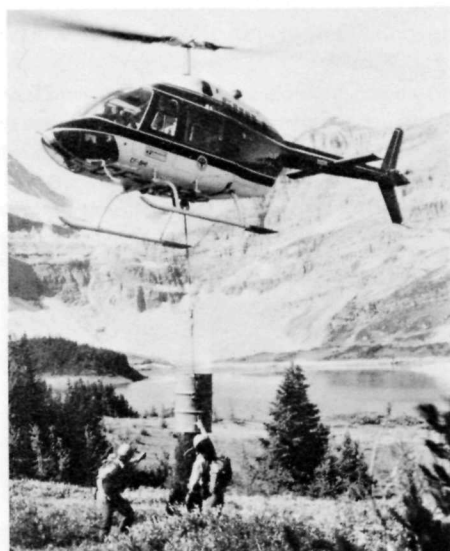
Gravelling mountain trails: one Ranger guides the helicopter pilot into position, then his partner releases the load of gravel.
