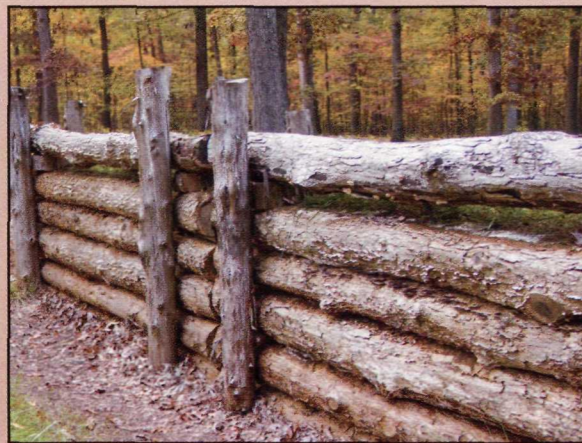
Based on written accounts and early postwar photos of Overland Campaign fortifications, this breastwork-reconstruction at Spotsylvania is shown from the defender's point of view. The "headlog" at top is elevated by design to offer a rifleman head-protection while standing in the trench and firing through the gap below.
