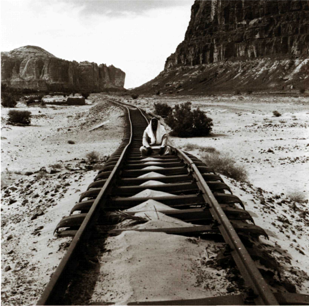
Railroad builders on the arid Arabian Peninsula faced terrain not unlike that of much of the American West; this is the old Hijaz line north of Medina.
