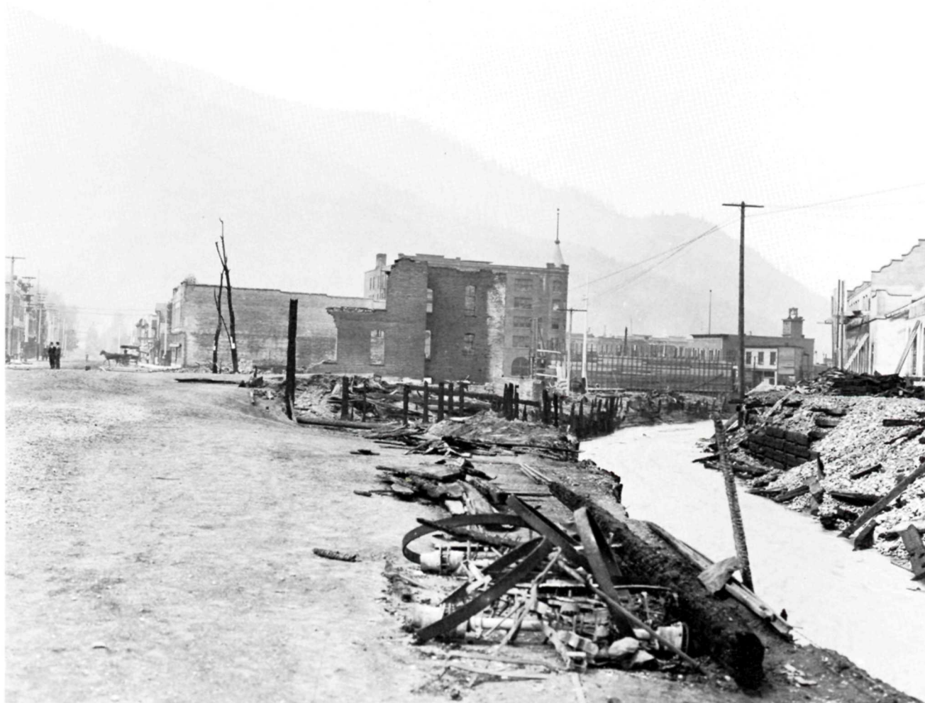
A row of brick buildings and a change in wind direction enabled the people of Wallace, Idaho, finally to turn aside the 1910 fire, but only after the railroad depot, a hotel, an iron foundry, two breweries, and 150 homes had burned.
