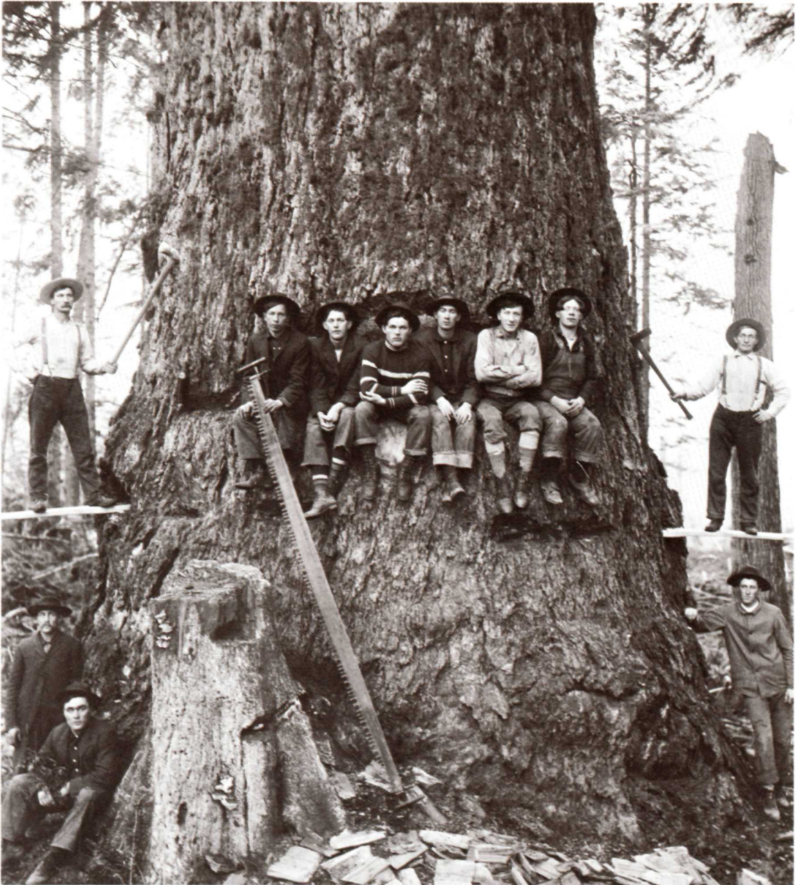
Six young loggers sit comfortably in the undercut of a seventeen-foot-diameter Douglas fir. Fallers flanking them have had to cut new notches to support their precarious springboard perches as they chopped deeper into the tree. Like most of the views on these pages, this Kinsey photograph dates from the first third of the twentieth century.
