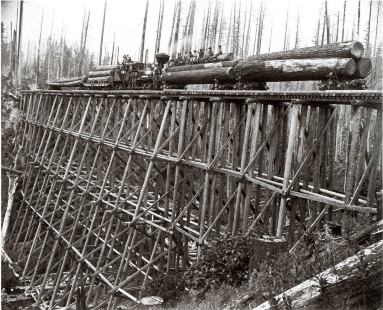
Lofty trestles for the log trains required enormous amounts of timber for construction and were among the loggers' most impressive monuments. Here a train poises nearly one hundred feet above a ravine for Kinsey's camera.
