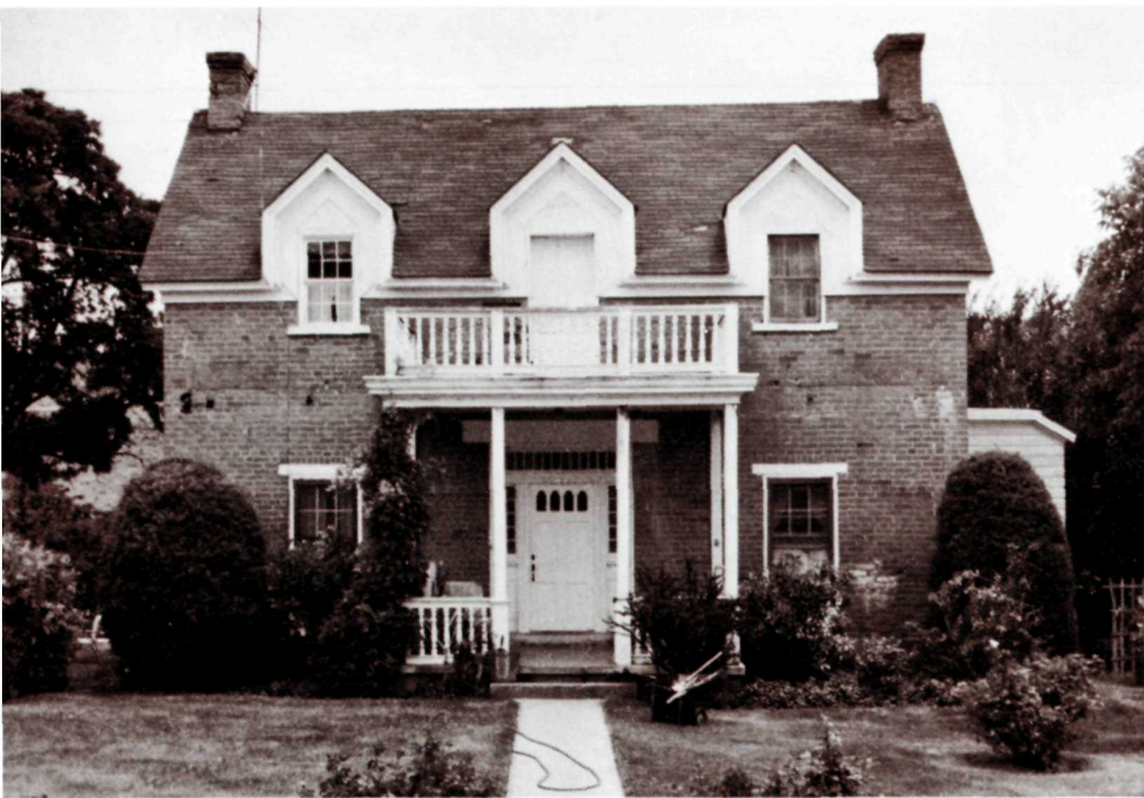
The William Stirling house in Leeds, built in about 1876, is the most famous example of a home built with "Dixie dormers"—an effect achieved by carrying the cornice up and around the dormer windows and eaves in a continuous line. Only about eight or nine houses with Dixie dormers remain in southern Utah; all are located in the region around St. George.
