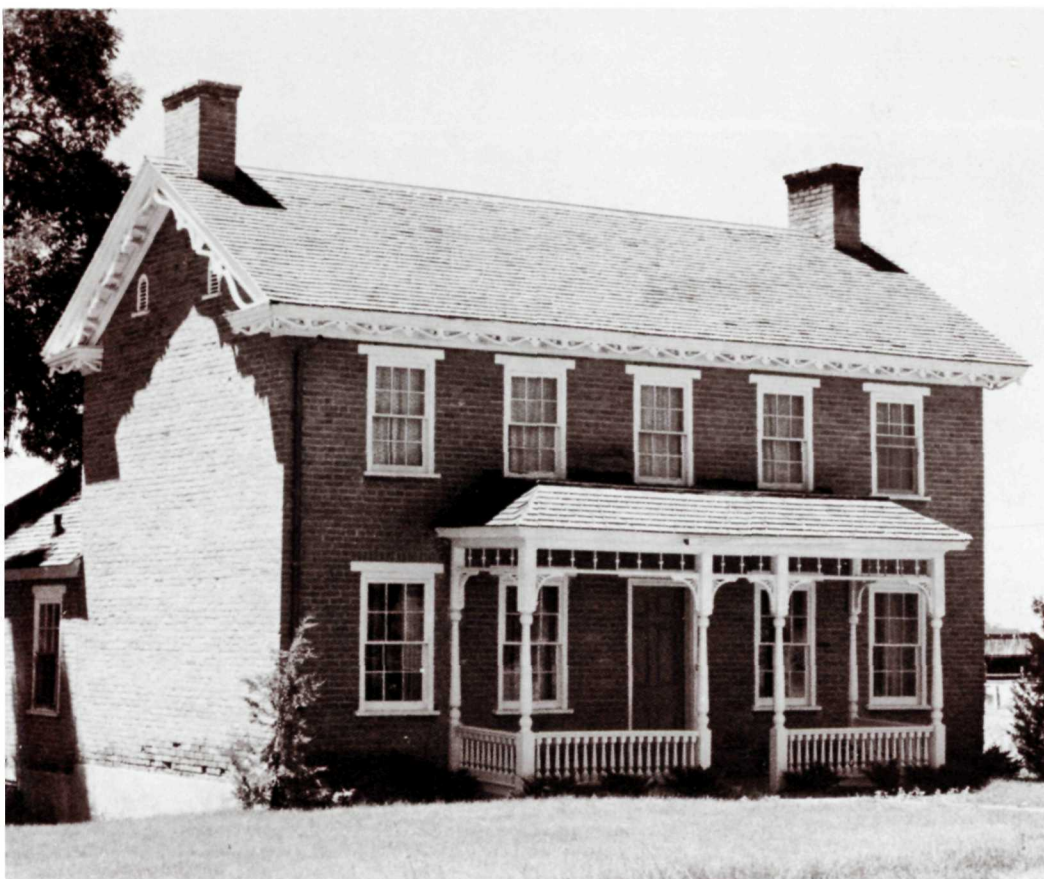
David Riley Stevens, the first bishop of the Latter-day Saints ward in Holden, Utah, built his two-story red brick home there in 1872. A lovely example of the standard "Nauvoo" or central-hall plan, it is decorated conservatively with white trim, some gingerbread, and two beehive-shaped attic ventilators.
