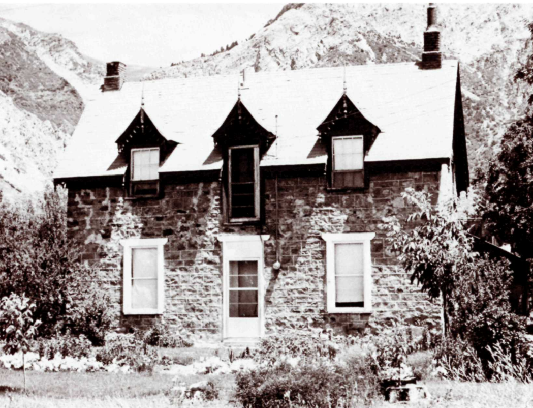
The Omer Call house in Willard, built in 1861, is located in a northern Utah region of stone houses in quality and number unmatched elsewhere in the state. The most prominent builder was the Welsh-Mormon immigrant stonemason Shadrach Jones, who built this home, his own larger one in Willard, and others throughout northern Utah. The basic design of this central-hall house is pure Utah, but the trim is faintly "alpine."
