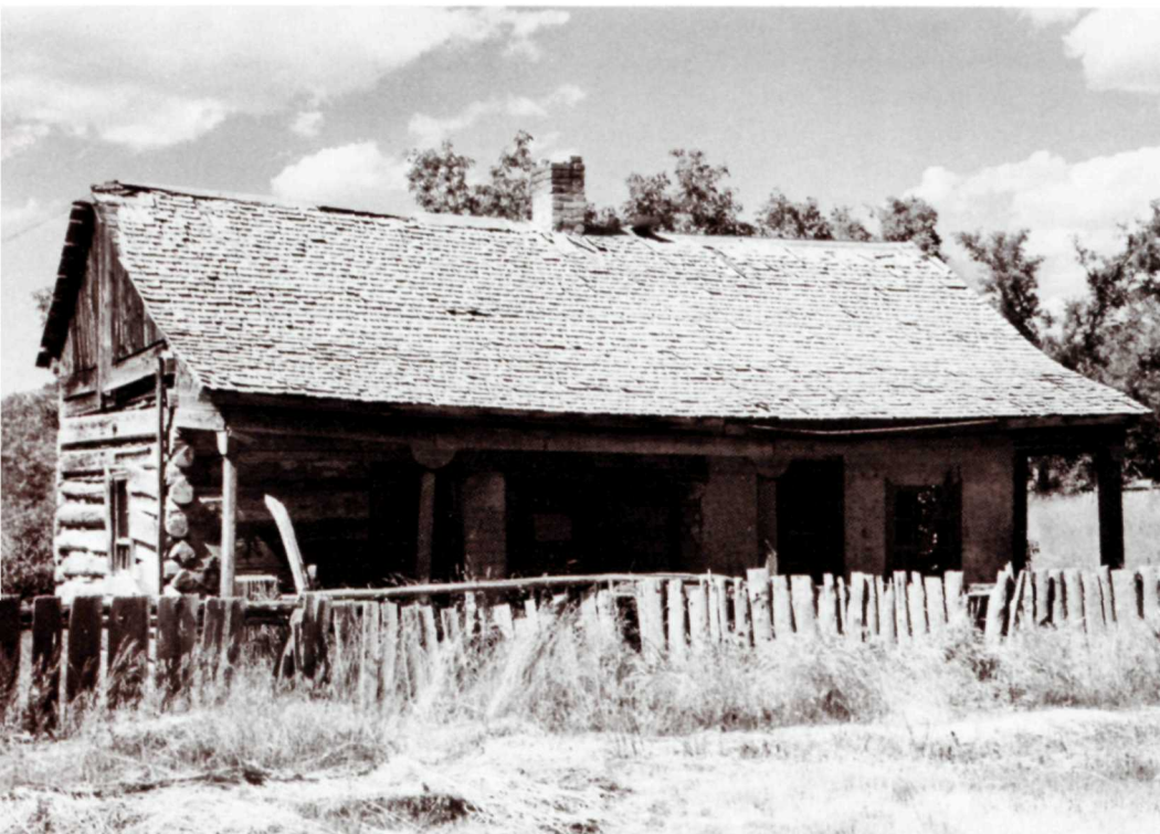
This house in Spring City, Utah, illustrates the transition from log to adobe construction. The left half was originally a square log cabin with V-notched logs; the right-hand half, probably added later along with the porch, was built from adobe bricks. In front of the house is a typical "Mormon fence" put together with unpainted, uneven, vertical boards.
