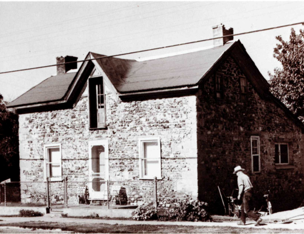
This small house of coursed rubble with solid quoins is in Toquerville, one of the oldest Mormon settlements in southern Utah. The upstairs door leading nowhere is a typical Utah puzzle. (Some people suggest such curiosities were intended to facilitate the moving of furniture or as places to shake out bedding.)
