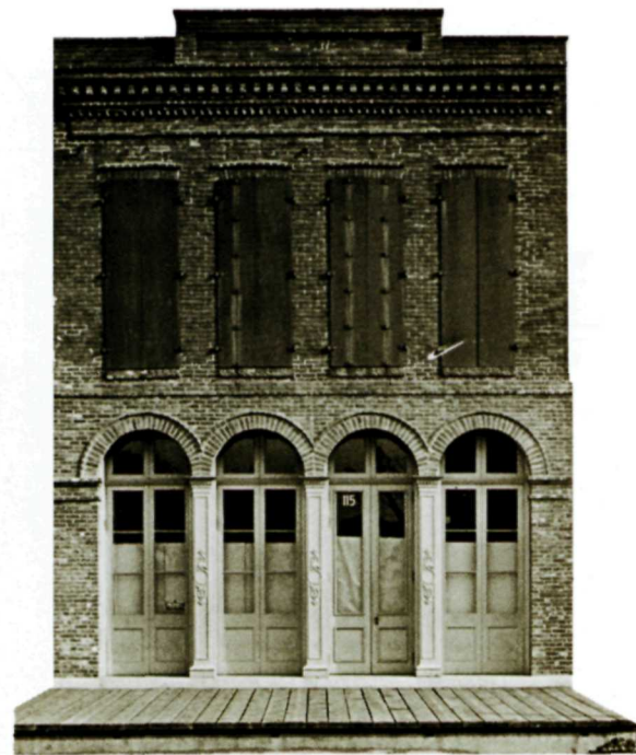
DINGLEY SPICE MILL, 115 I STREET COFFEE AND SPICE MILL; BUILT IN 1853 (PRESENT STRUCTURE IS A RECONSTRUCTION) SCHEDULED TO HOUSE A PORTION OF THE STATE RAILROAD MUSEUM
