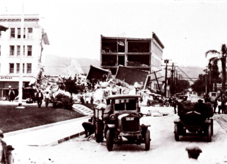
Southern California is as much subject to earth tremors as is the northern half of the state. This view shows some of the wreckage in Santa Barbara's business district that resulted from the shocks of June 29, 1925.
