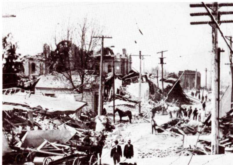
Most heavily-hit town in the April 18, 1906, California earthquake was Santa Rosa, fifty miles north of San Francisco. As in the larger city, devastation from shocks was followed by fire. Santa Rosa is located some distance from the San Andreas fault, and the severe damage was blamed in large part on poorly constructed buildings.
