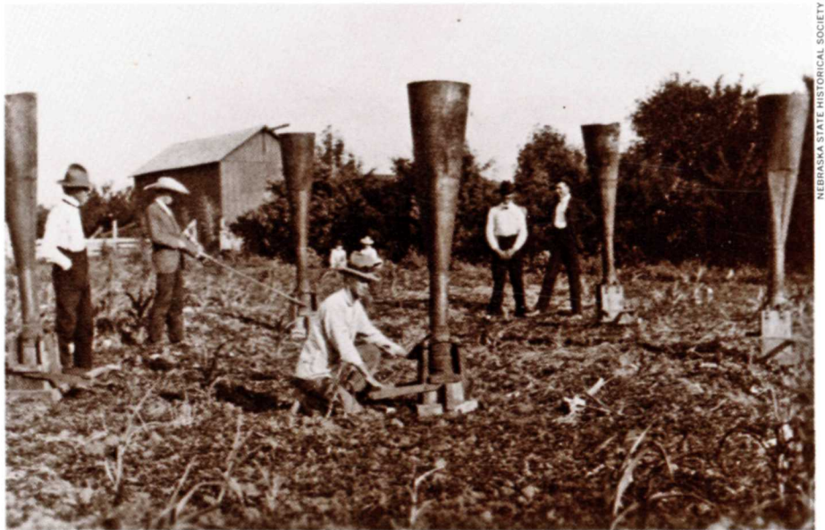
THE WRIGHT GASEOUS GENERATION EQUIPMENT IN OPERATION
