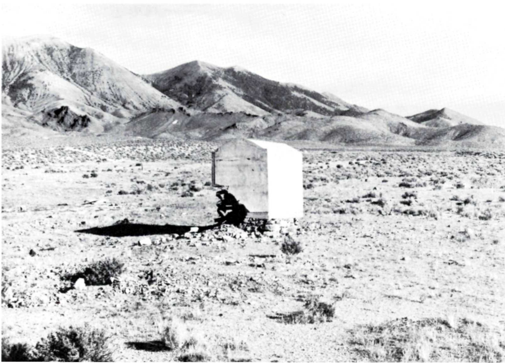
Fairview, 1968: Except for this cement bank vault and the surrounding caved-in cellars, the town of Fairview has disappeared from the face of the earth.
