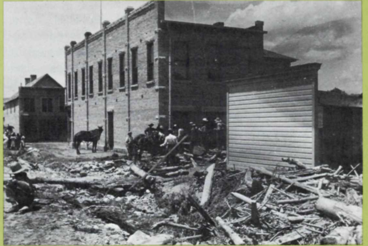
For a good many years this was almost an annual occurrence in Manti, Utah, situated on an alluvial slope at the mouth of Manti Canyon.
