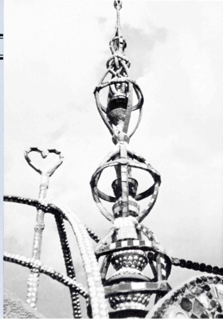
Detail of the towers, showing seashells, bottles, and plates used in the construction.
