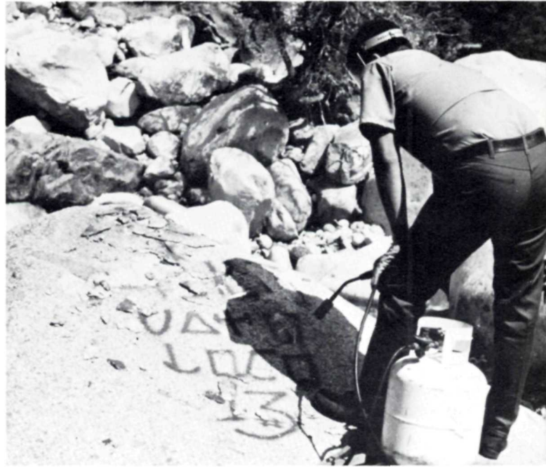
Vandals' moment of fun with spray paint takes workers a half-hour to erase with acetylene torches.
