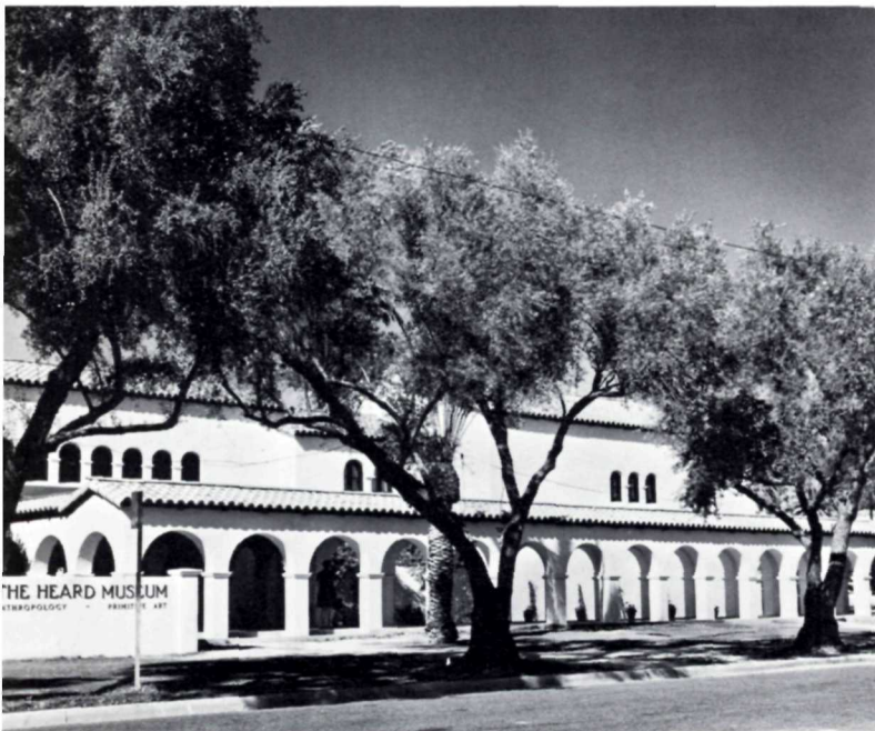
The Heard Museum of Phoenix revives the tiled roofs and simple arches of the Mission style.
