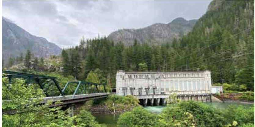
The entire flow of the Skagit River re-emerges here after running through a two mile underground tunnel at Seattle City Light's Gorge Powerhouse just above Newhalem. The Gorge hydropower project "de-waters" the Skagit here, permanently blocking migratory salmon. —PHIL FENNER PHOTO
