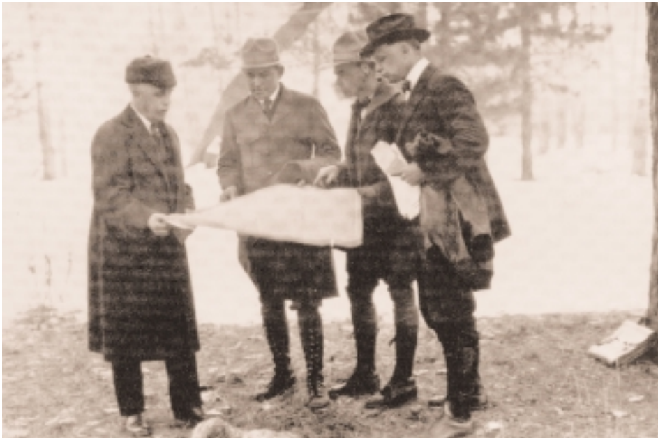
In November 1922, James Greenleaf (far left) of the federal Commission of Fine Arts conferred with Daniel Hull (middle left) and others on the plans for the new village in Yosemite Valley. Courtesy NPS Historic Photography Collection
