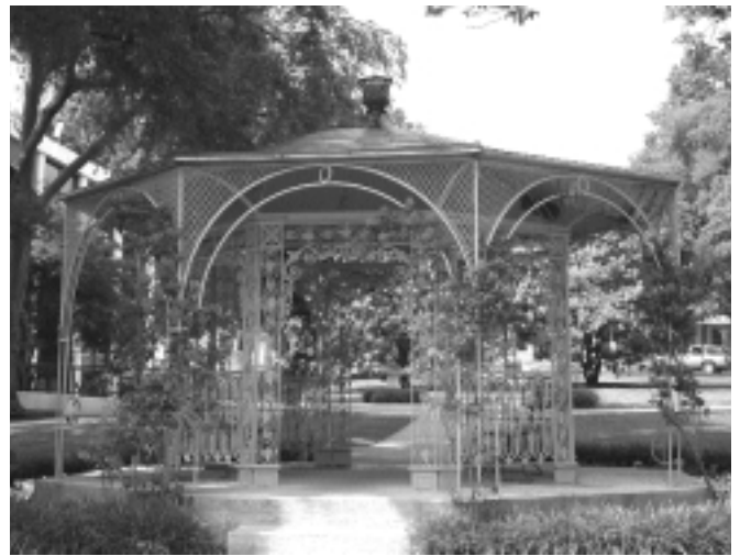
Cast and wrought iron gazebo at center of gardens, circa 1853-1861, made by Janes, Kirtland and Co. of New York. Gardens may have been designed by estate owner, Joseph Acklen. Courtesy Belmont University (Belmont Mansion Association).
