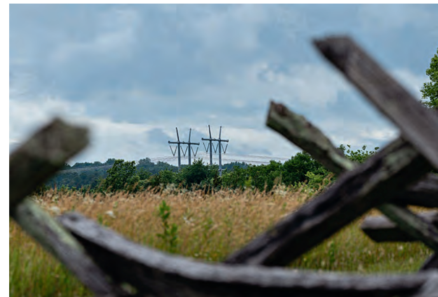
PROponents of the digital gateway reference these transmission towers, which march along the park's western boundary, to support their argument that the area is no longer rural.
