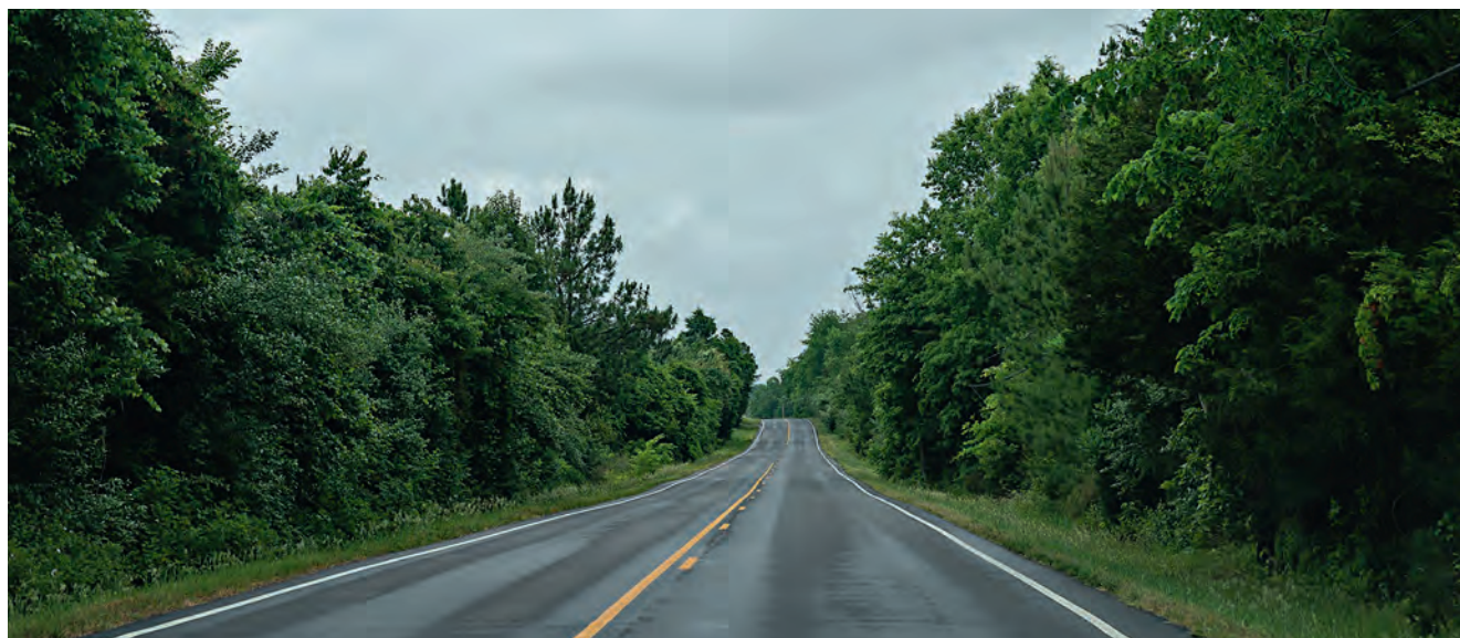
A DATA CENTER COMPLEX in Sterling, Virginia, complete with industrial cooling equipment and water tanks (top). Above: Under the current digital gateway plan, Pageland Lane (pictured) would turn into a four-lane, divided road, with data centers and substations along its length. According to an early viewshed analysis done by the county, any buildings over 35 feet tall would be visible from key points within the park. “Will people still choose to go there as much?” asked longtime park advocate Ann Bennett. “I don’t know.”
