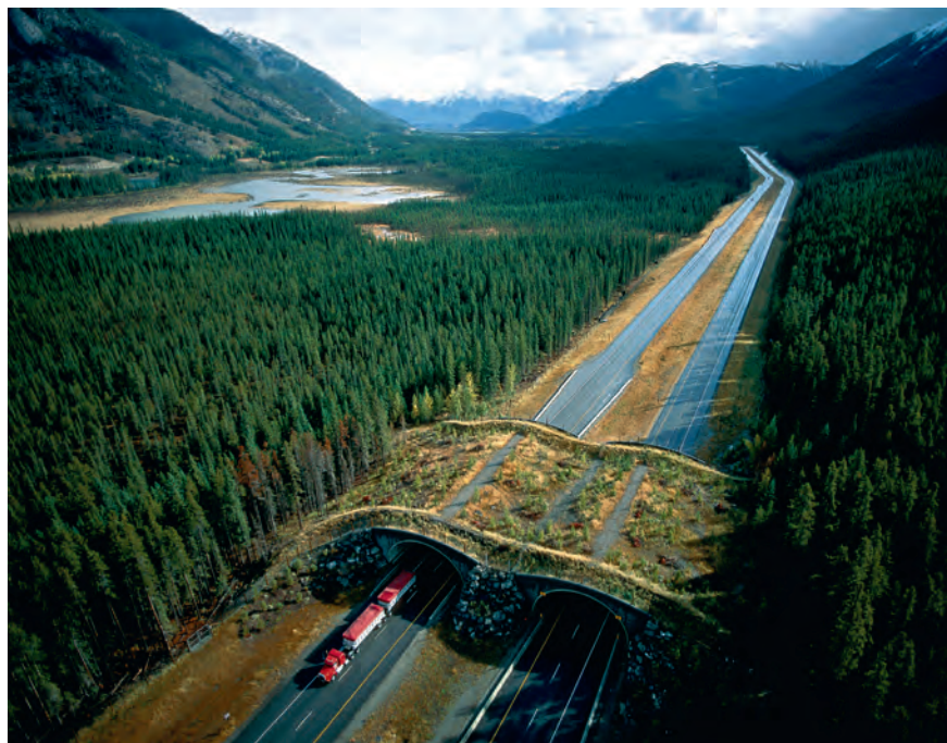
A WILDLIFE CROSSING in Canada's Banff National Park. The park boasts six such overpasses and 38 underpasses, as well as some 50 miles of fencing along the Trans-Canada Highway. Since their installation, these safety features have reduced wildlife-vehicle collisions in the park by more than 80%.
