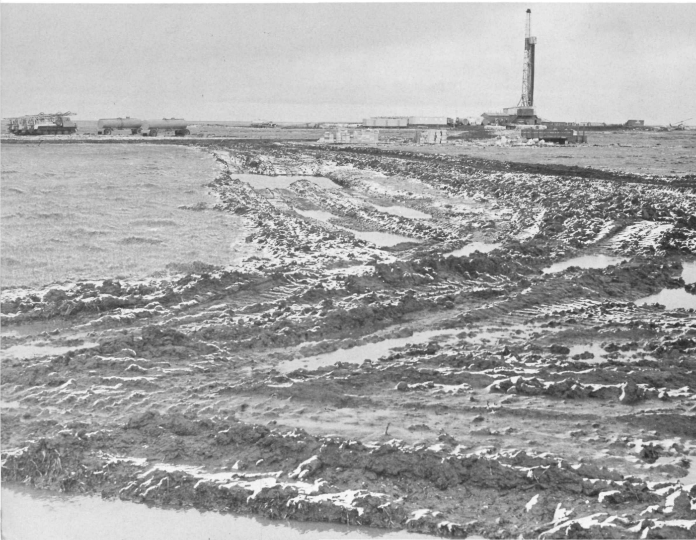
An insufficient layer of gravel in road construction resulted in thawing of the permafrost and severe degradation of the tundra at this well site at Pt. Storkensen operated by Pease-Hamilton.
