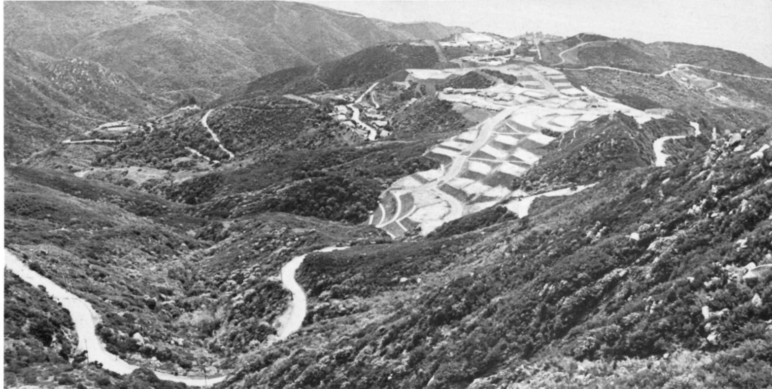
Despite efforts to curtail real estate development within the Santa Monica National Recreation Area, residential development is proceeding there with alarming speed and disastrous consequences for the environment.
