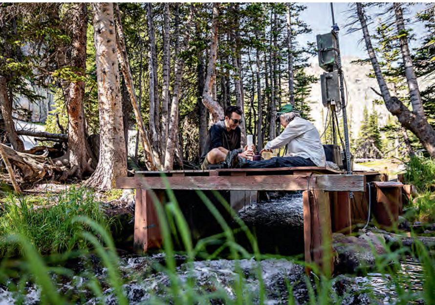
WEINMANN AND BARON working on the platform built over The Loch's outlet, where water exits the watershed.
