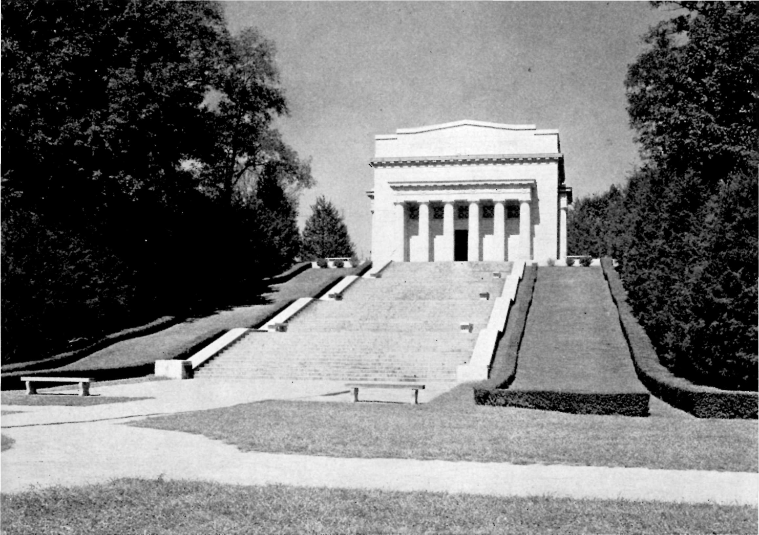
The Memorial Building, within which is preserved the traditional Abraham Lincoln birthplace cabin. This structure of classic simplicity is built of Connecticut pink granite and Tennessee marble
