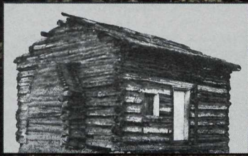
The cabin before its placement inside the Memorial Building.
