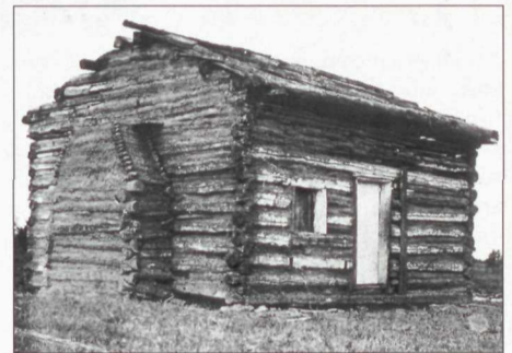
The cabin before its placement inside the Memorial Building. NPS
