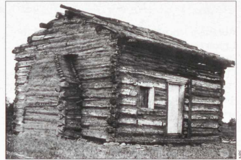
The cabin before its placement inside the Memorial Building.
