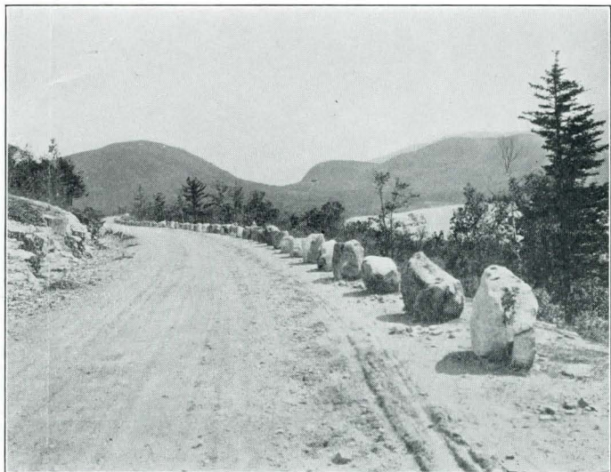
Section of Cadillac Mountain Road Lafayette National Park
