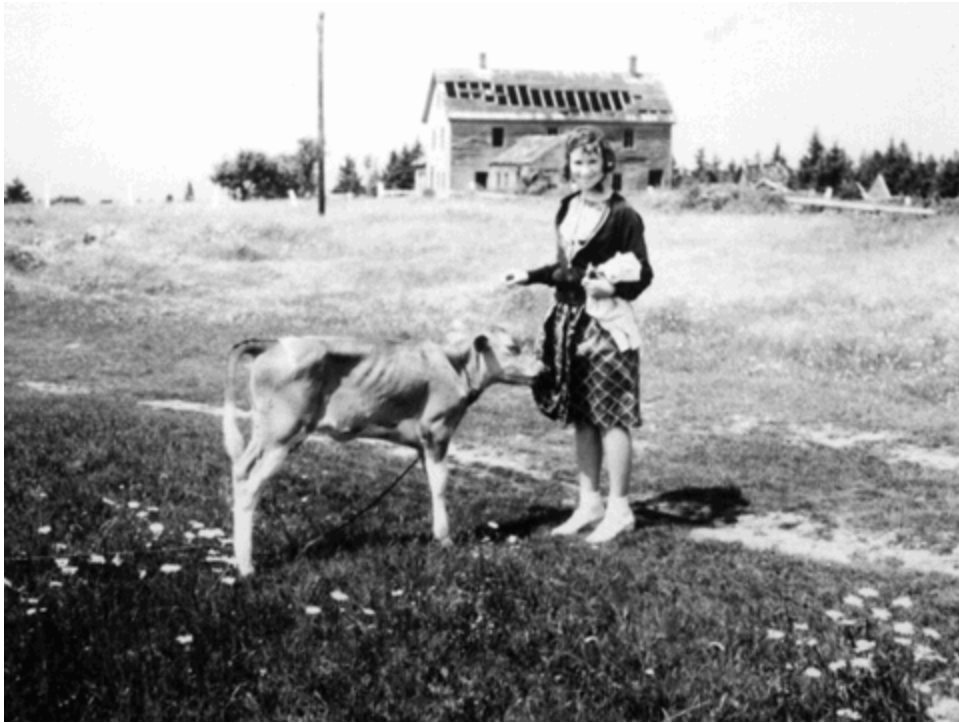
Figure 13. View looking north of the deteriorating Joseph Gilley/Charles A. Gilley house, with the house in more ruinous condition and the barn already removed or collapsed, ca. 1940s. (Acadia National Park Archives)
