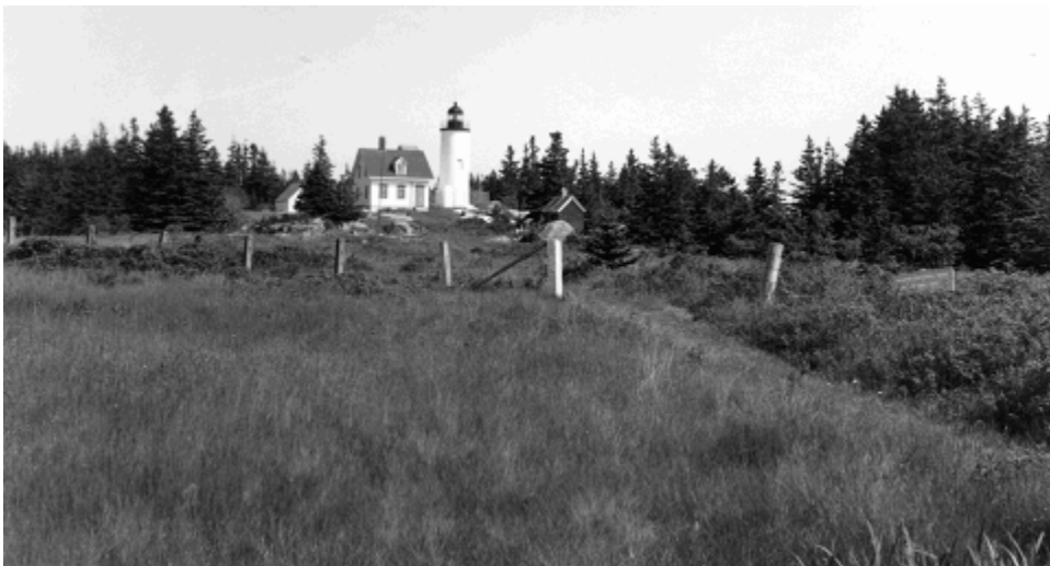
Figure 15. View south in ca.1958 of (from left) paint locker, keeper's house, watchtower (behind house), light tower (passage gone, fence up), and oil house (tanks gone). More trees since ca.1937 (Fig 8). (No. 0633, Acadia National Park Archives)
