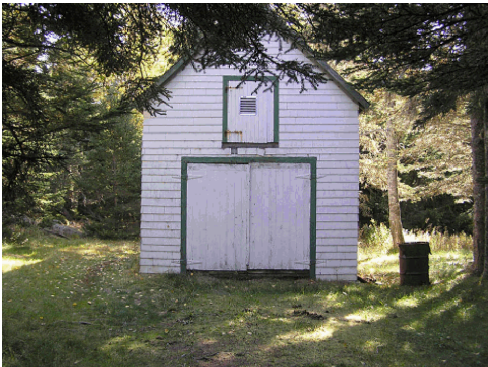
Figure 25. View looking south at the front of the ca.1905 fuel house, also known as the garage. (OCLP 2008)
