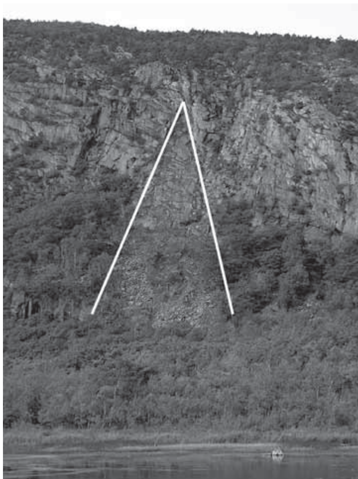
Rock slide caused by earthquake. Photo by NPS/Karen Anderson.
