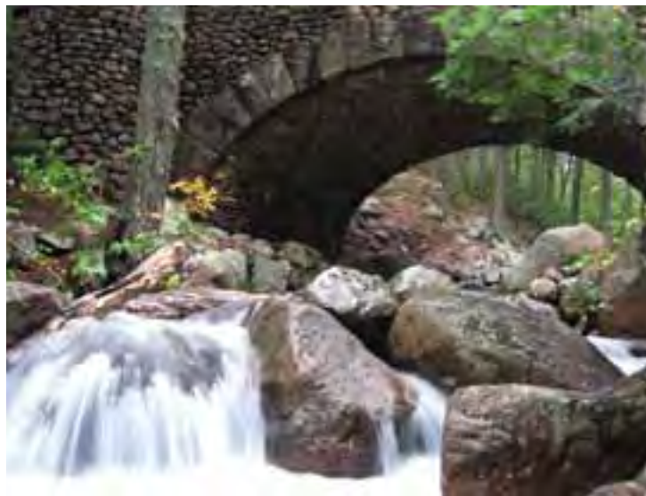
Cobblestone Bridge after a fall rain
