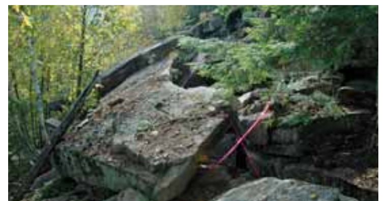
A granite slab blocks Homans Path. Photo by NPS/Kevin Cochary.
