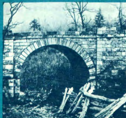
Skew Arch Bridge
