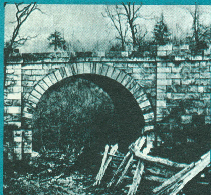
Skew Arch Bridge
