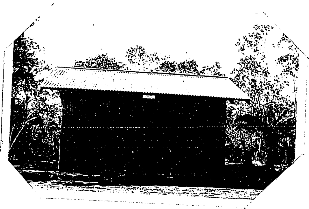
New Gasoline and Oil Building
