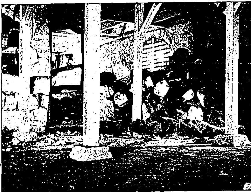
Collapse of partitions in cellar of Puuwaawaa Ranch House resulting from earthquake damage October 5, 1929. Note the wooden posts diagonally braced and footed in concrete, which saved the house when the cellar walls gave way.
