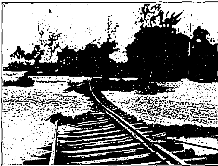
Railroad embankment washed down by tidal wave between Hilo and Kuhio Wharf February 3, 1923. The major wave at Hilo was the third noticed visually, and the waters rose over 20 feet in places damaging wooden houses and wharves. Damage was done also at Kahului in Maui. Photo Morihiro.
