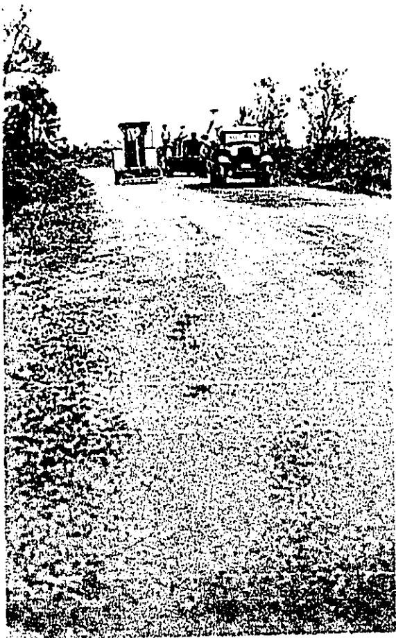
Resurfacing park highway at Kan entrance, job 526 force account
