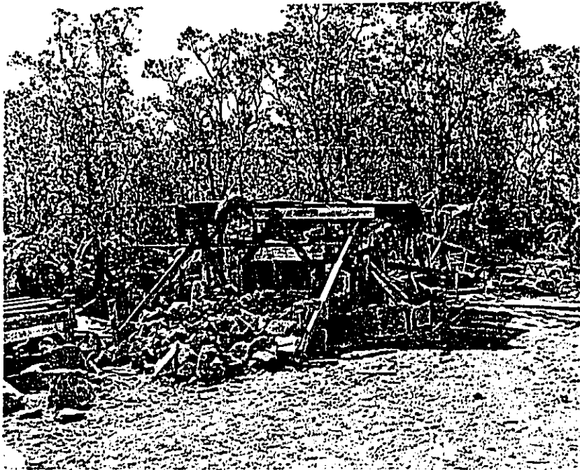
Incinerator - progress photo. CCC Project
