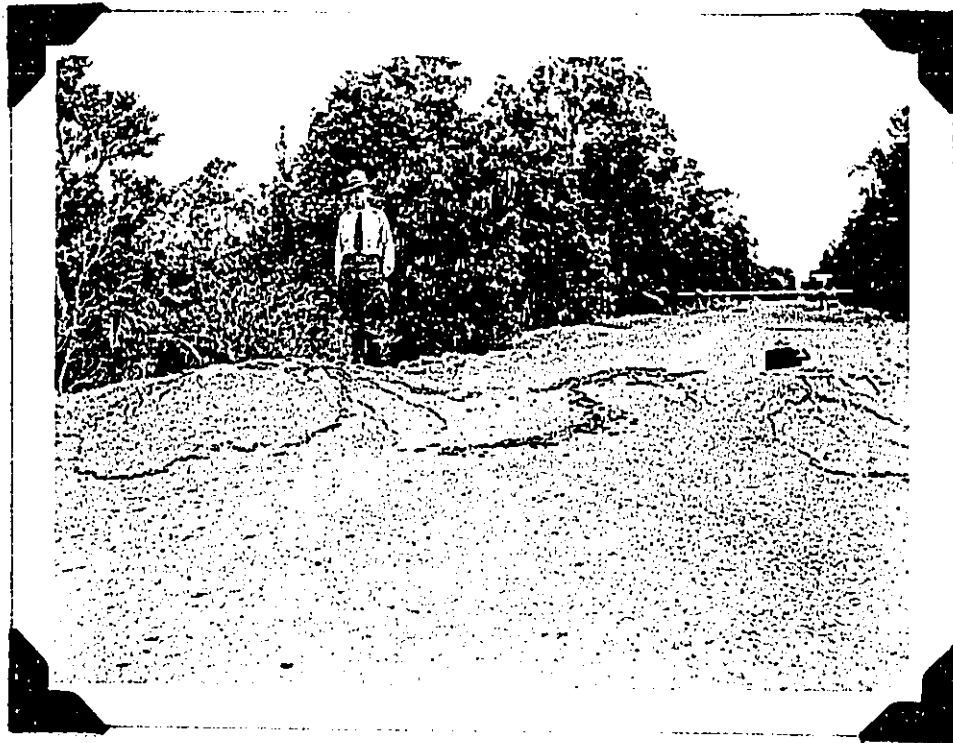
Nos. 2 and 3 - Two views along Chain-of-Craters road showing humping of road accelerated during spasm of earthquakes on August 8.
