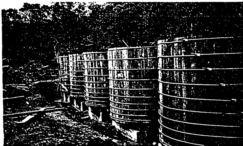
Above - Water storage supply at new CCC Camp - Tanks removed from old camp and set on concrete foundations
