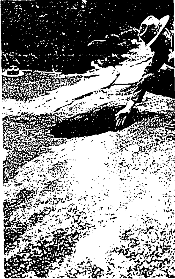
Hole that opened in Chain-of-Craters road near Pauahi crater underneath rear wheel of ranger's car as he drove over the spot.
