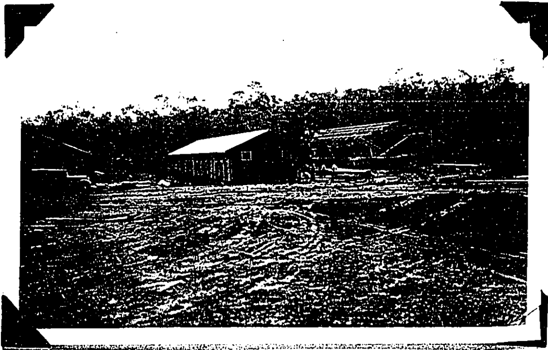
No. 5 - Construction new CCC camp. Two bunkhouses about complete and hospital framing going up. Photo by Pope, March 10
