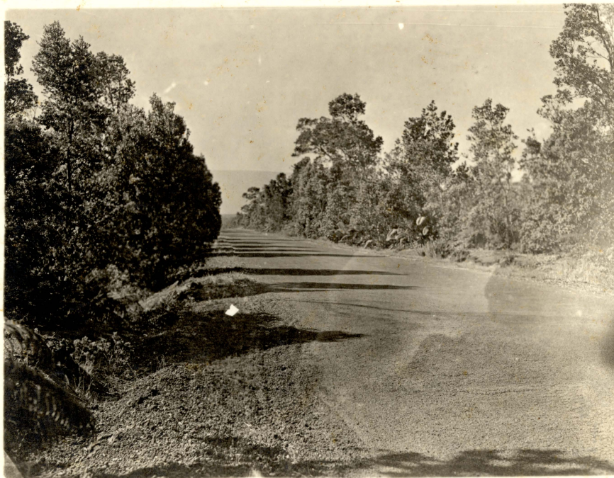
One of the "Humps" on Chain of Craters Road that is growing, Mauna Loa showing faintly in back ground
