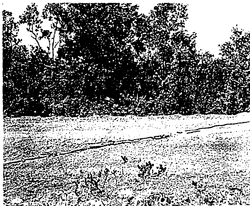
No. 8. One of 18 or more cracks which developed across roadway during earthquake spasm beginning May 28.
