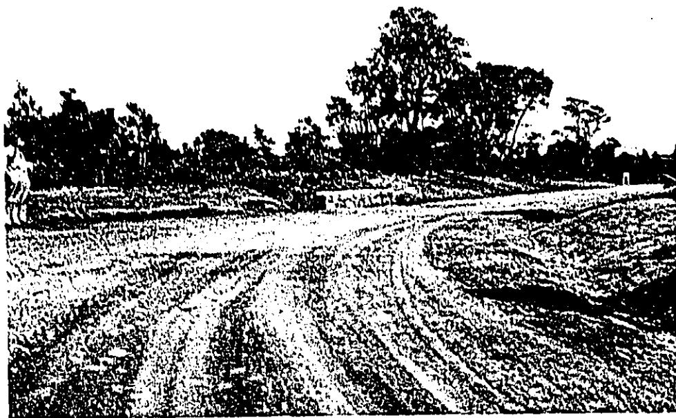
Above - Entrance to new road to theatre at Kilauea Military Camp constructed by CCC
