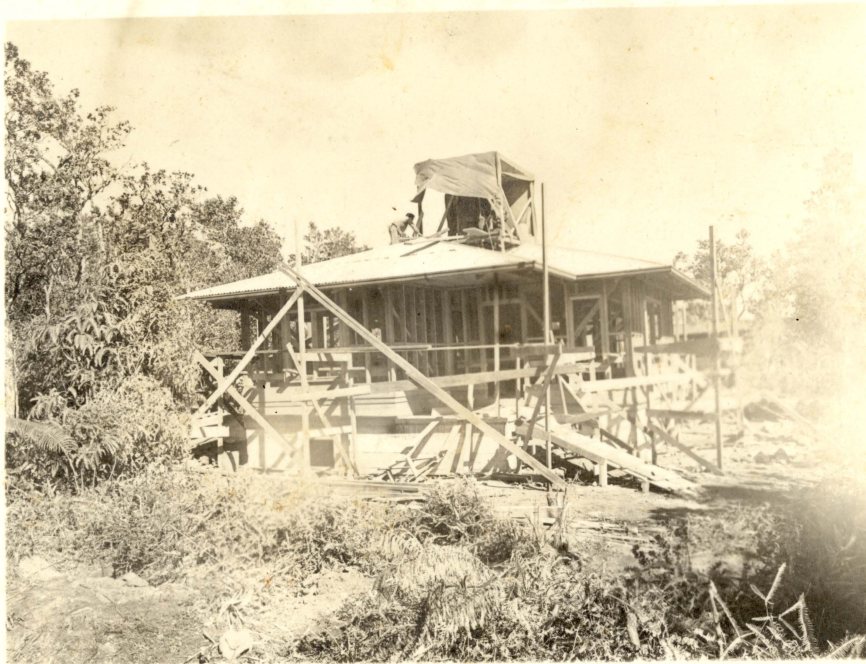
Cottage #3 CCC job about 50% Complete, Photo Dec. 15th
