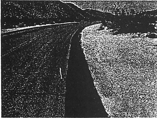
Asphalt strip along damaged section of road edge
