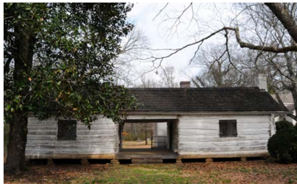
MTSU researchers visited the little-known John P. Hickman House, a “dogtrot” style building in Lauderdale County, Alabama.
