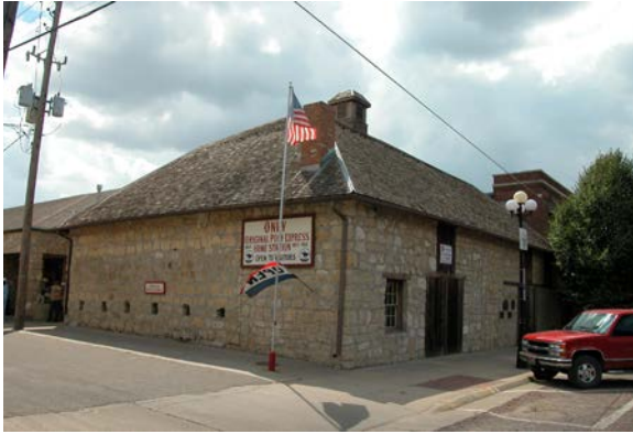
The Marysville (Kansas) Pony Express barn. One of only a smattering of Pony Express barns or stables still standing, NPS staff visited the site to survey needed structural repairs.
