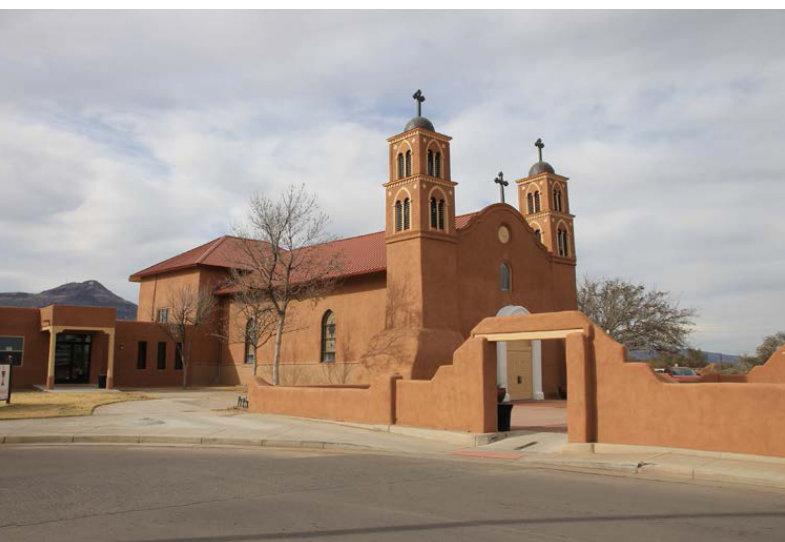
San Miguel Church, Socorro, NM, main façade and south side with sacristy (left).
