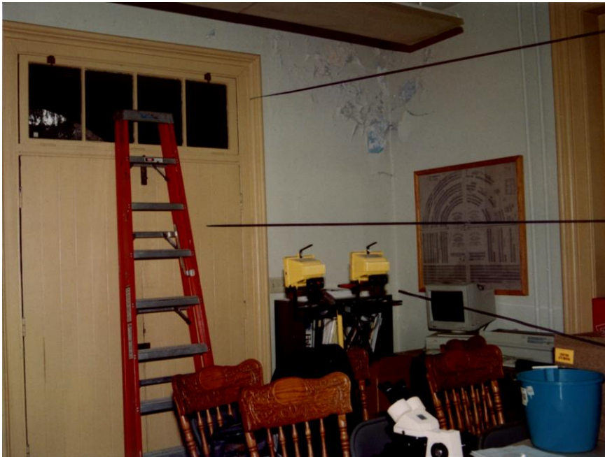
Photo 5. Office, Room 101. East wall.
