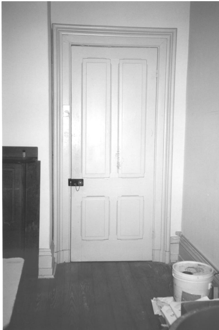
The door to the right (north) of the fireplace is typical of the interior paneled doors present throughout the building, although the doors are not all the same. This is an original door opening location. Note box lock on door. Photograph 1999, Robinson & Associates, Inc.
