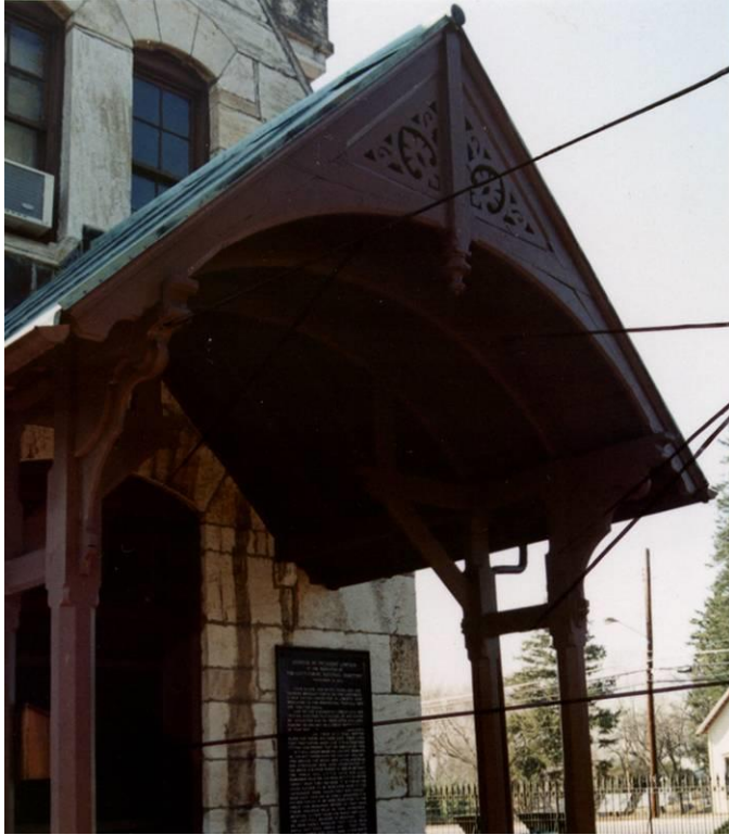
Photo 1. Exterior, east porch.
