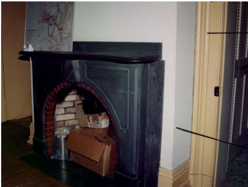
Photo 6: Office, Room 101. West wall.
