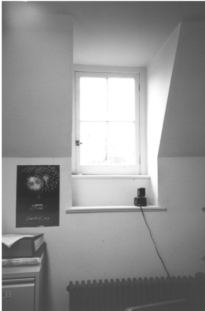
Typical windows on the second floor are in-swinging casements set into dormers. Note the canted walls that accommodate the hipped roof. Photograph 1999, Robinson & Associates, Inc.
