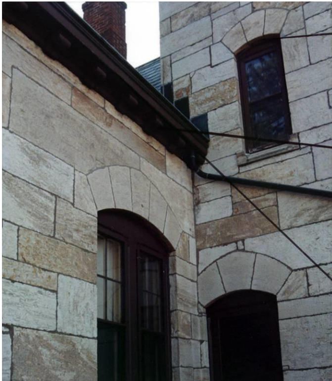
Photo 2. North door at east elevation.
