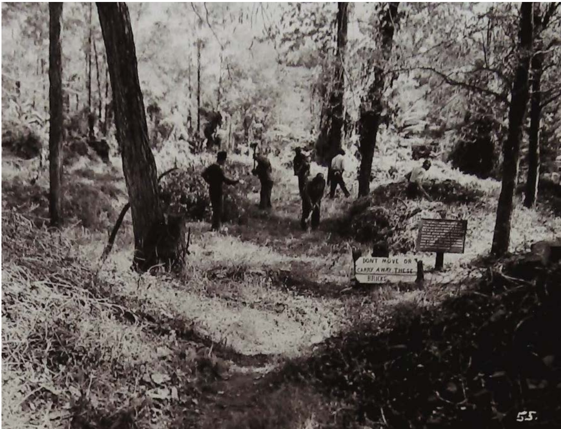
Figure 10. CCC enrollees clearing land at the site of the McLean House during September 1940. Note the iron War Department tablet in place and signage reading “DON’T MOVE OR CARRY AWAY THESE BRICKS.” “Administrative Files,” Box 1456, Entry P11, RG79, NACP.
