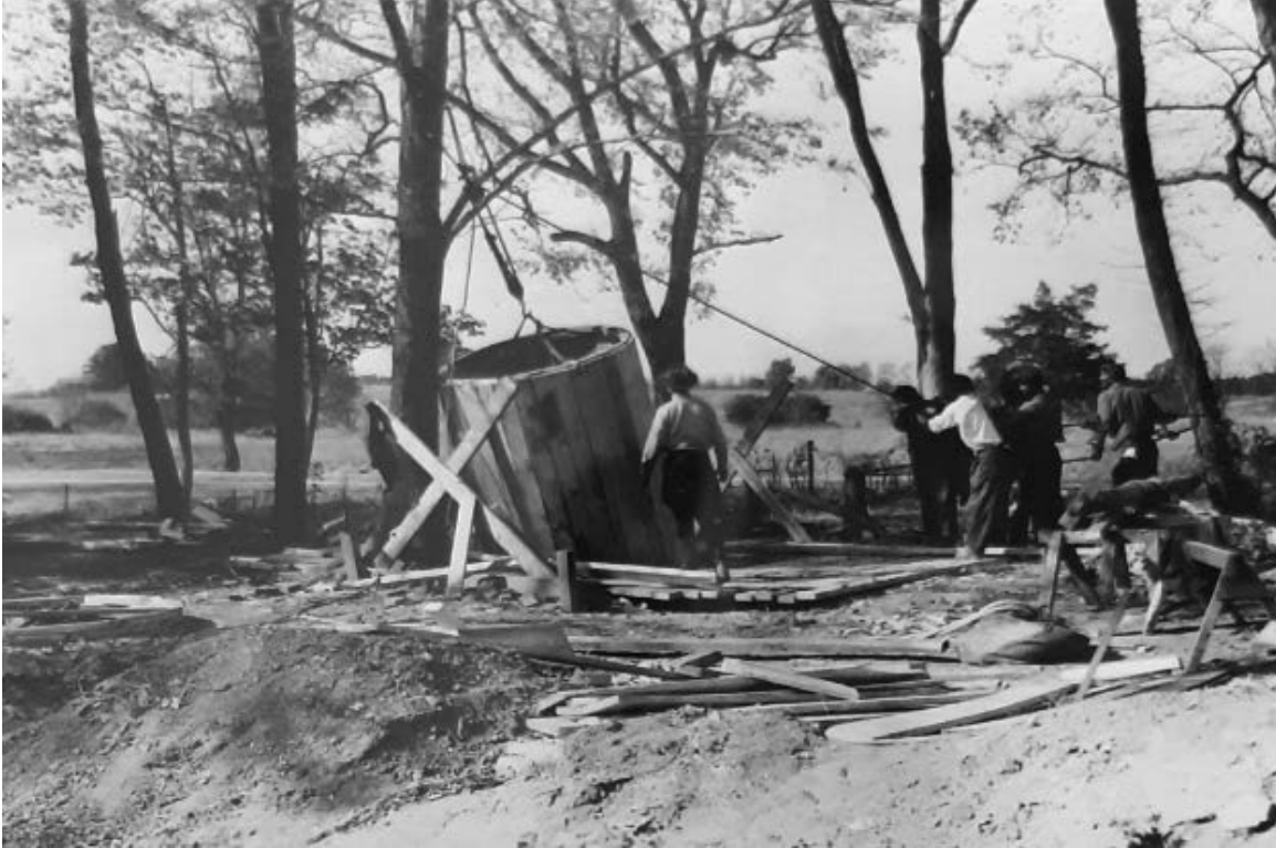
Figure 12. CCC enrollees installing wall shoring for the archaeological excavations of the McLean House well. SR, October 1941.
