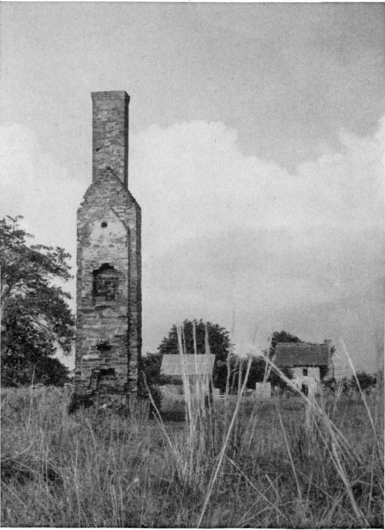
A view in old Appomattox Court House in 1940 at the time development work was started by the National Park Service.
