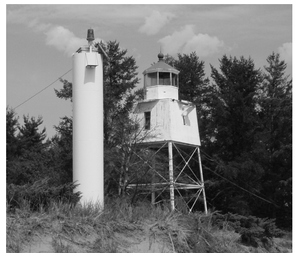
Top photo: LaPointe light tower and dock. Middle photo: Aerial photo by William Cronon Bottom photo: Chequamegon Point Lights, old and new.
